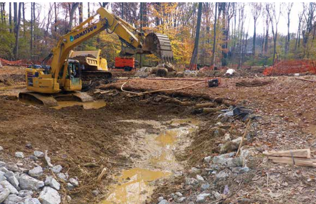
Fig. 1. A recent stream construction project at Upper Watts Branch Forest Preserve, City of Rockville, Maryland. Notice that the existing stream was completely destroyed to create an artificial floodplain by clearing the forested valley and raising the channel with tons of fill (sediment), tree trunks, and boulders. Photo by City of Rockville.
